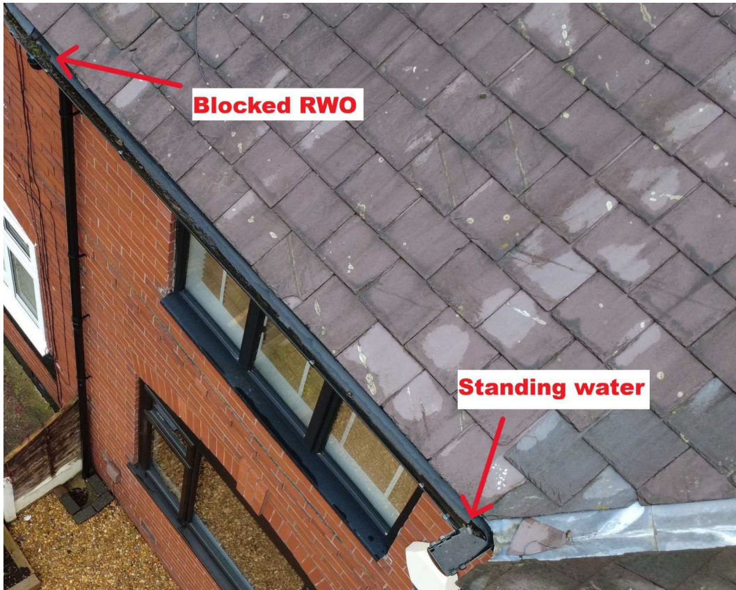
Main roof front guttering
