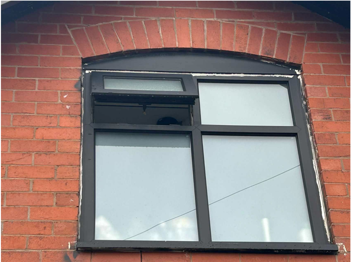
View to front bathroom window
