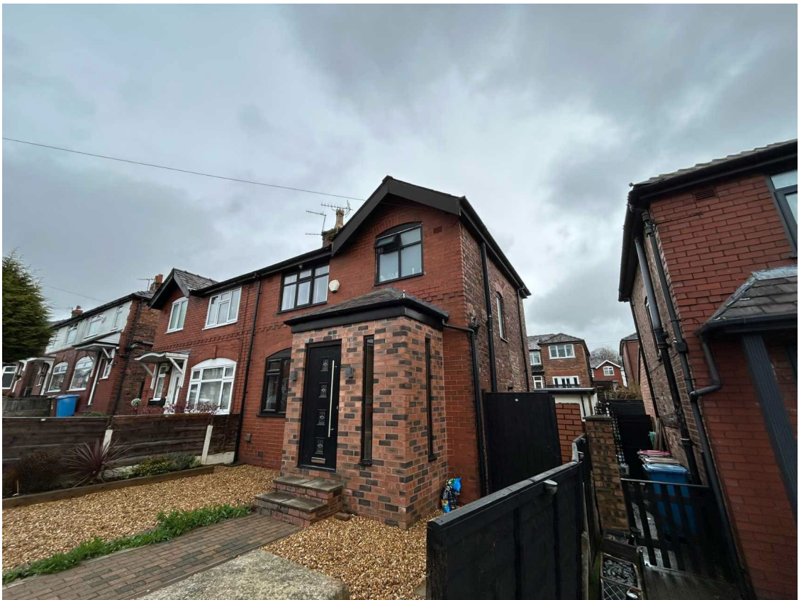
View to front from rhs
