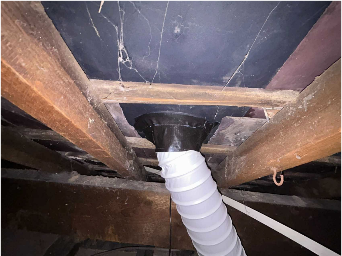
View to rear roof slope duct penetration
