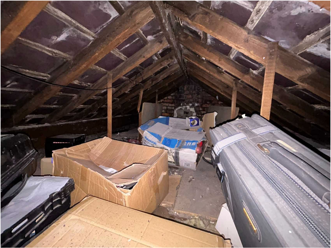
View to roofspace towards left hand side
