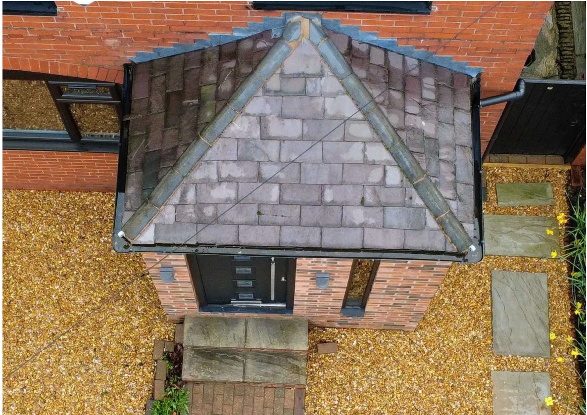
View to porch from above
