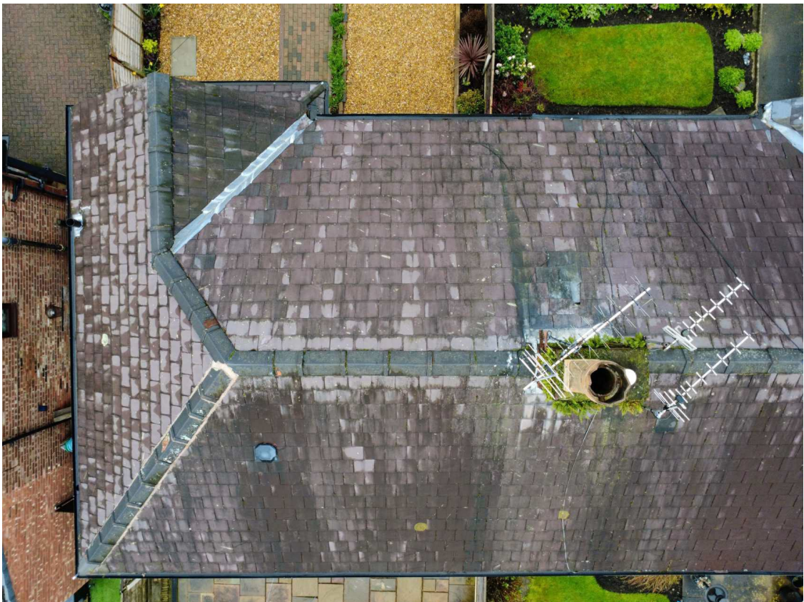
View to main roof from above
