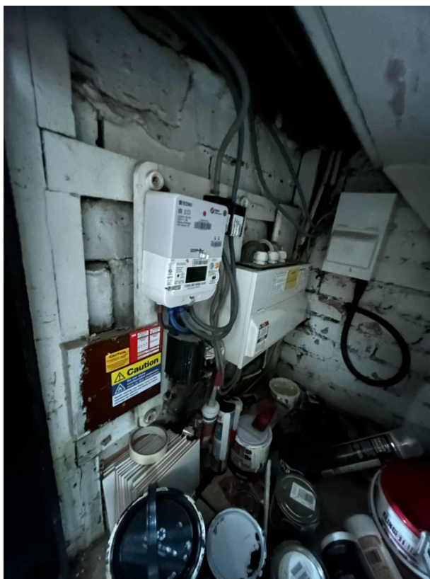
Electric meter/consumer unit
