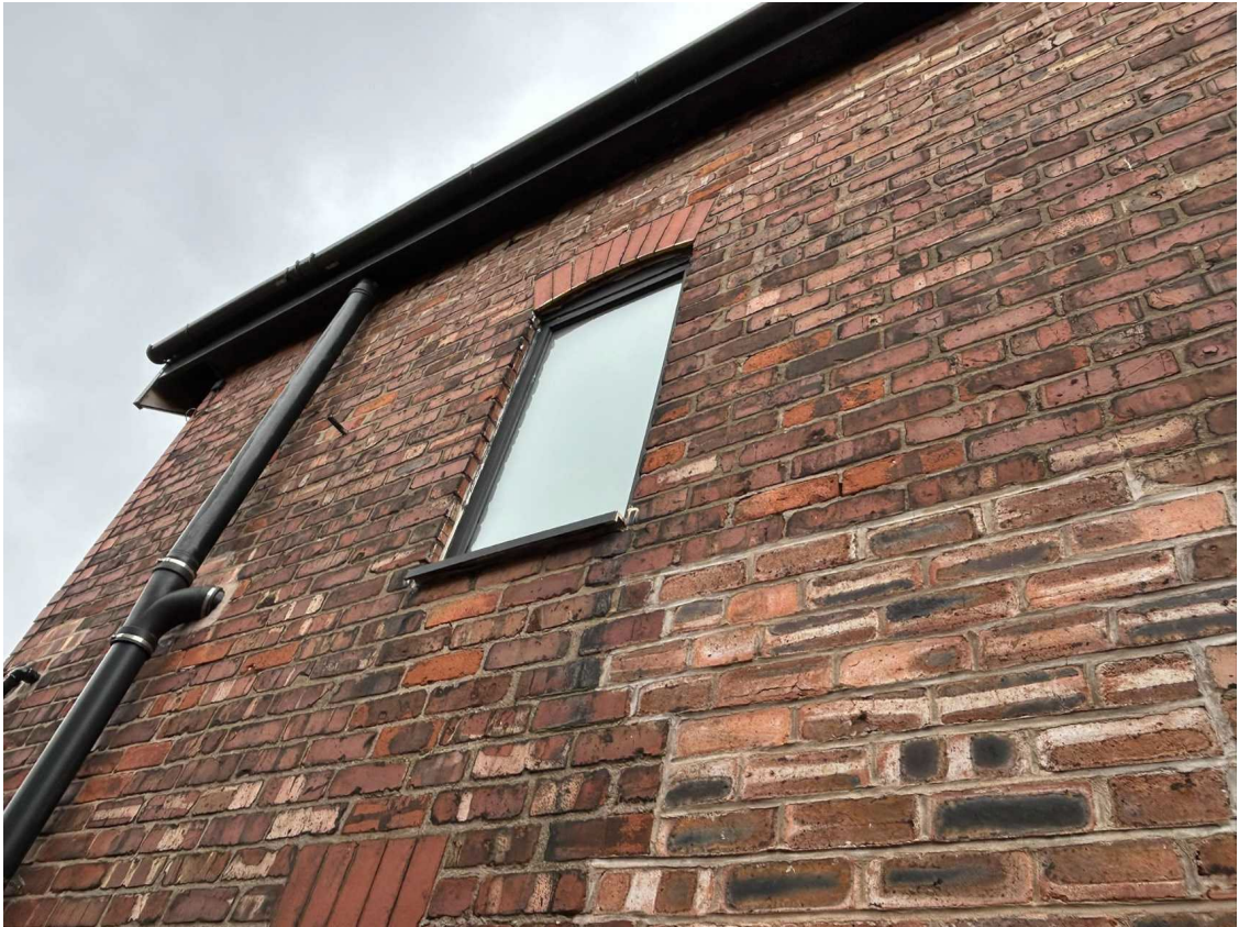
Soil pipe to the right-hand gable
