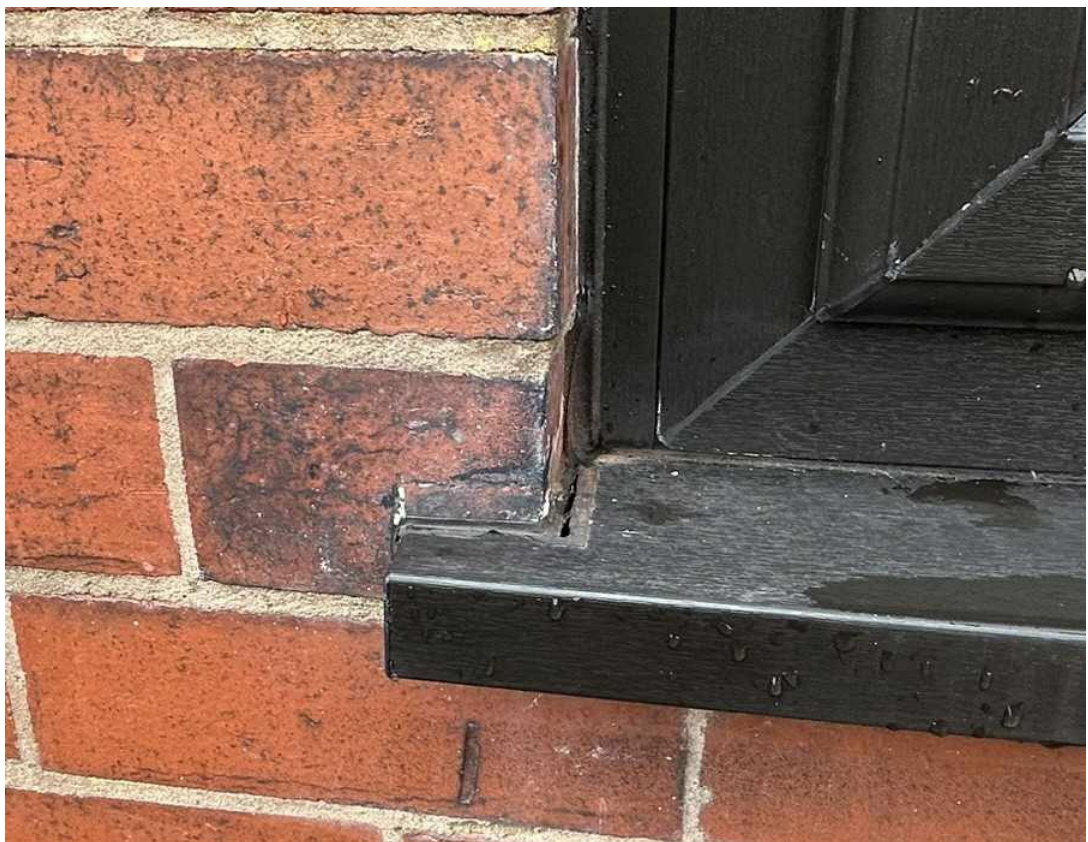
Gap to sealantt- lounge window
