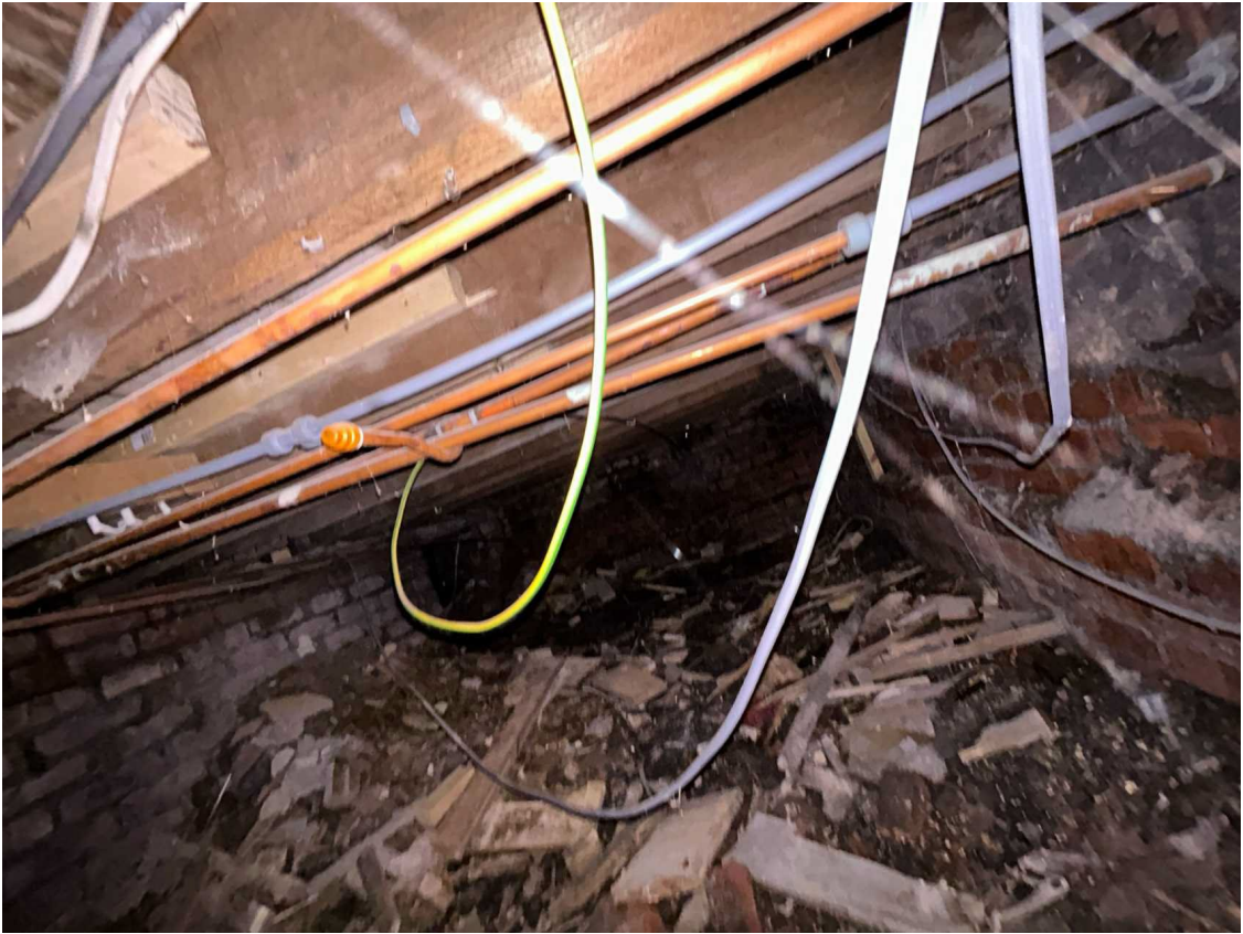
View to floor void
