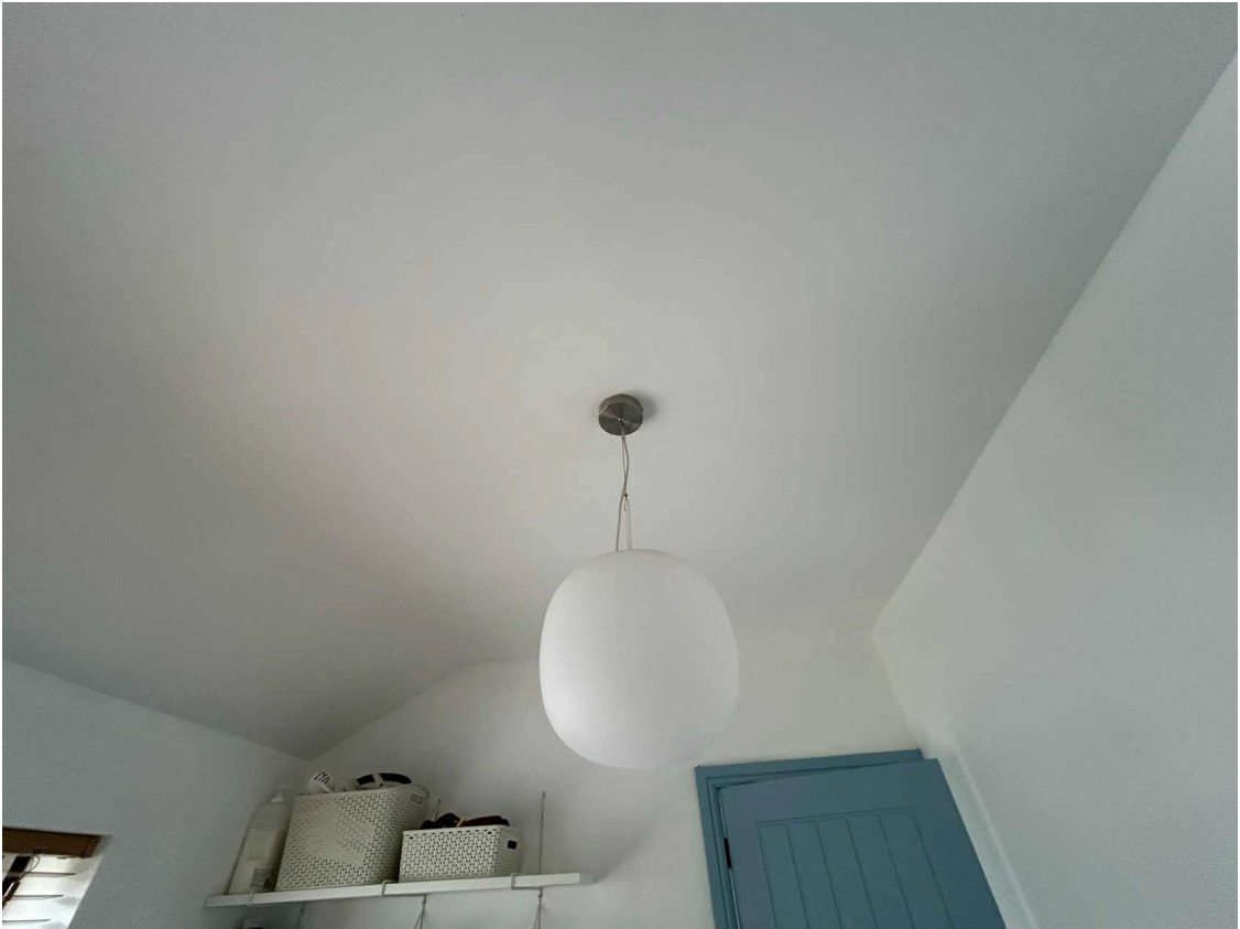
View to Bedroom 2 ceiling
