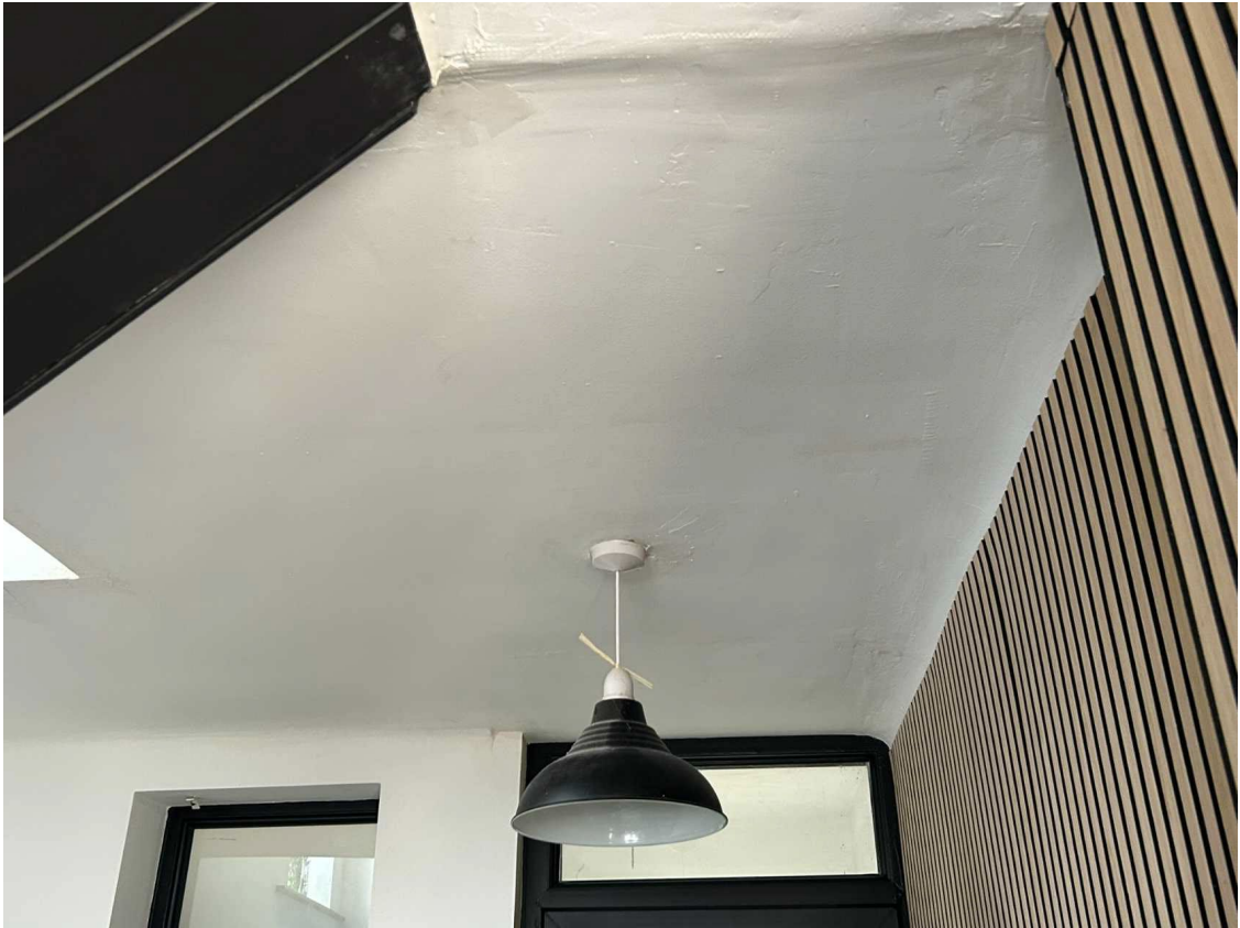
View to hallway ceiling
