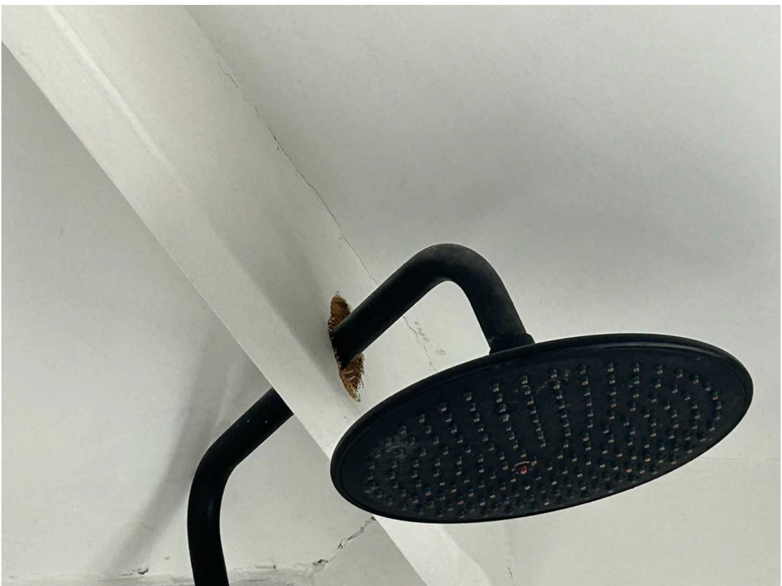
Shower fitting pass through, hip rafter
