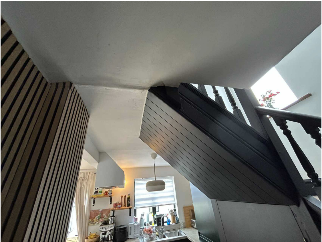
View to kitchen/hallway ceiling
