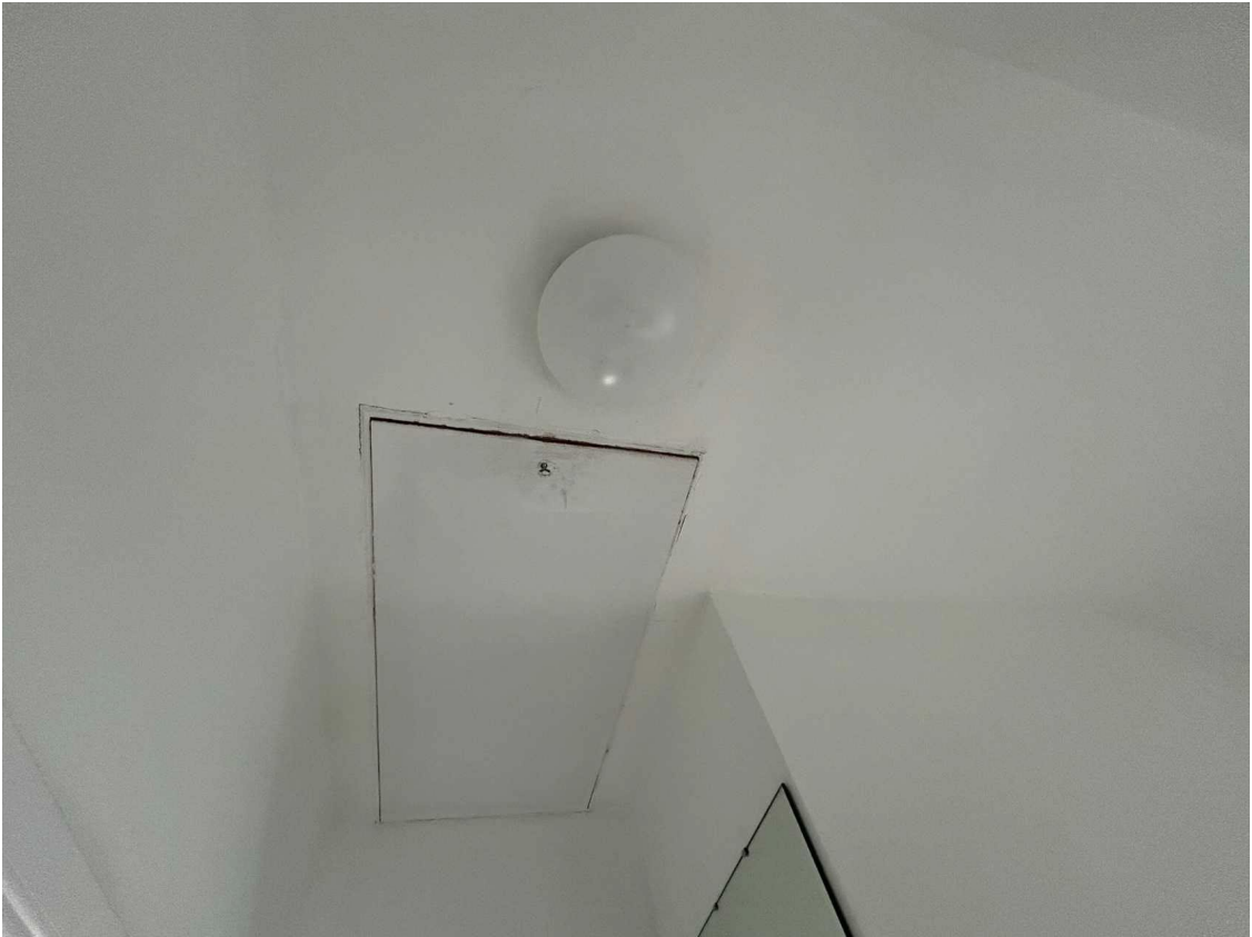
View to landing ceiling
