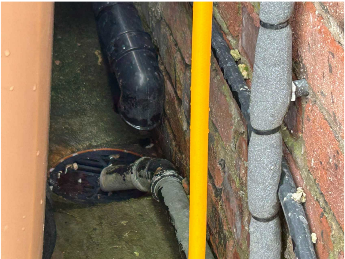
Waste pipes to the gully on the right hand side
