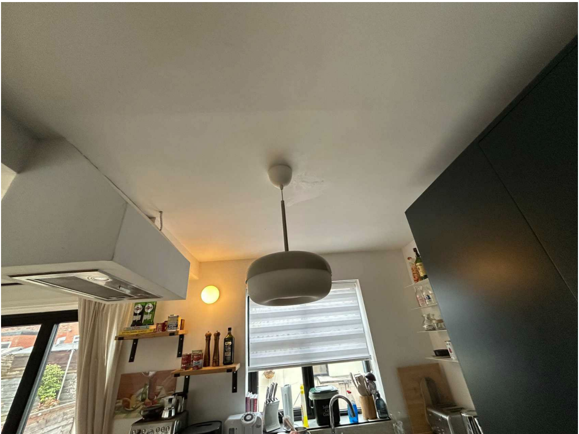
View to kitchen ceiling
