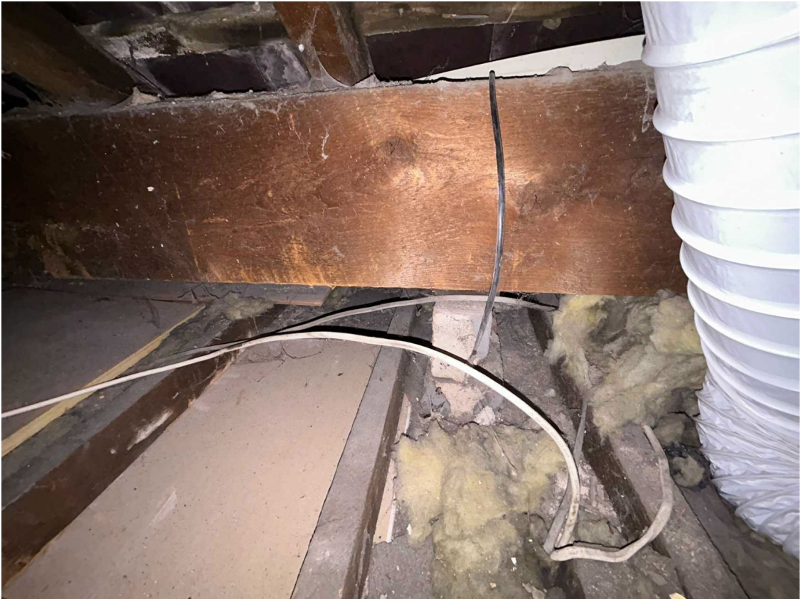
View to rear purlin supported of brick wall
