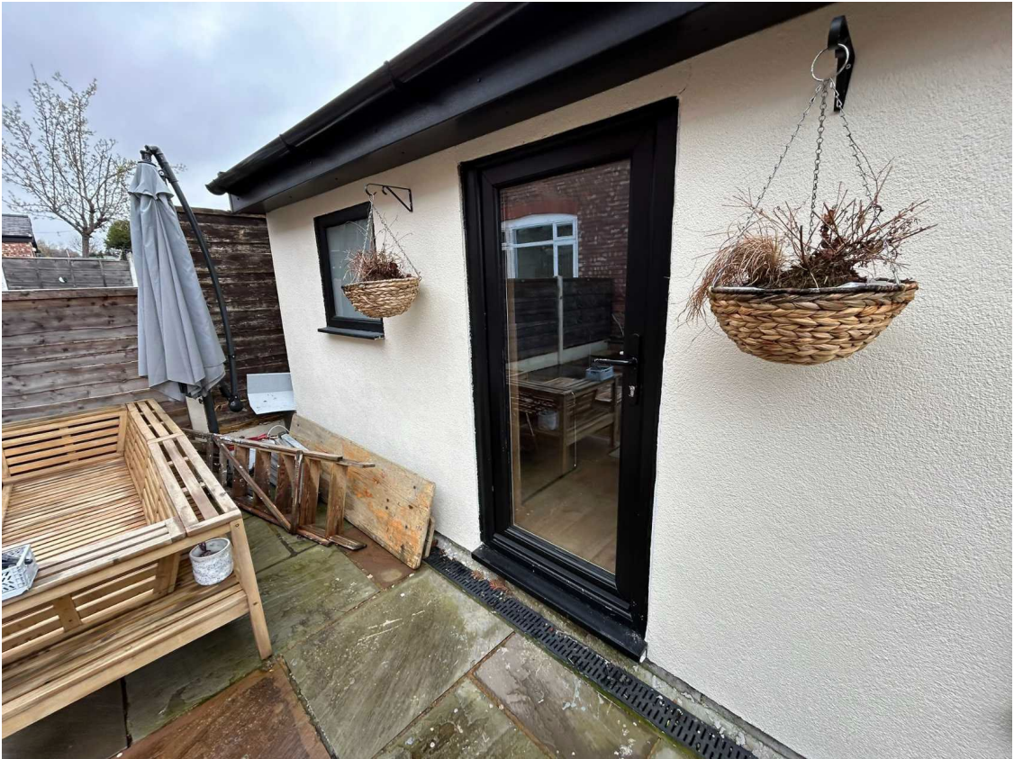
View to front of out-building
