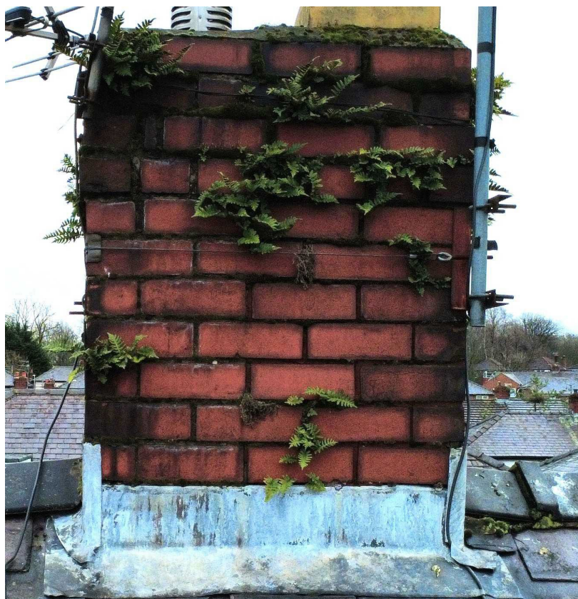
Chimney stack viewed from a drone at the front
