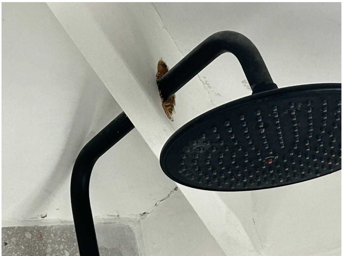
View to shower fitting- hole to hip rafter
