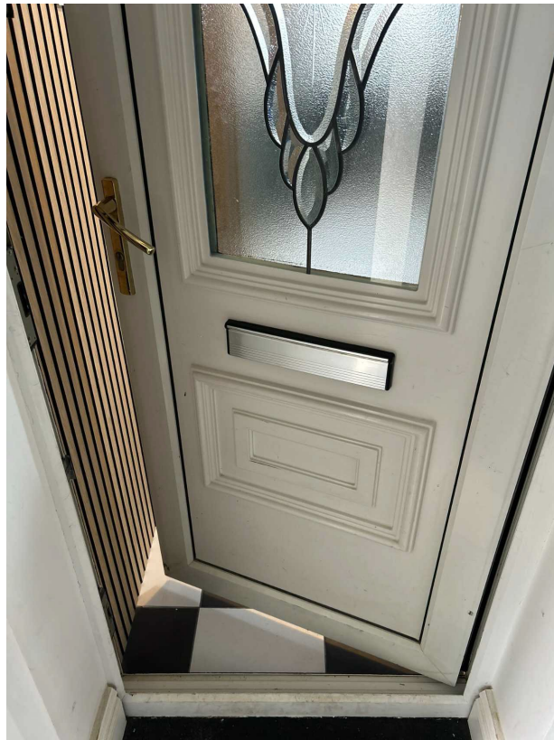
Upvc door from porch area
