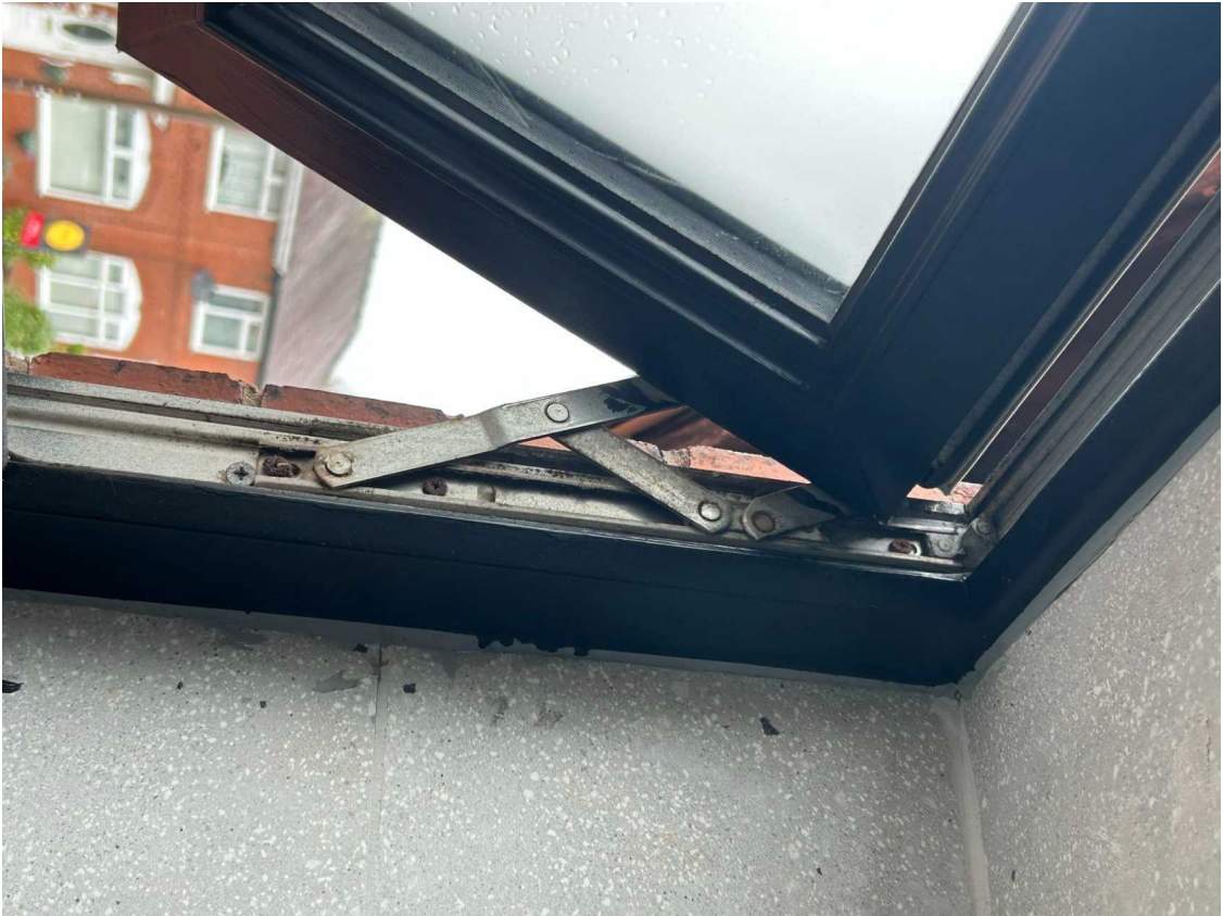
Ironmongery- corroded
