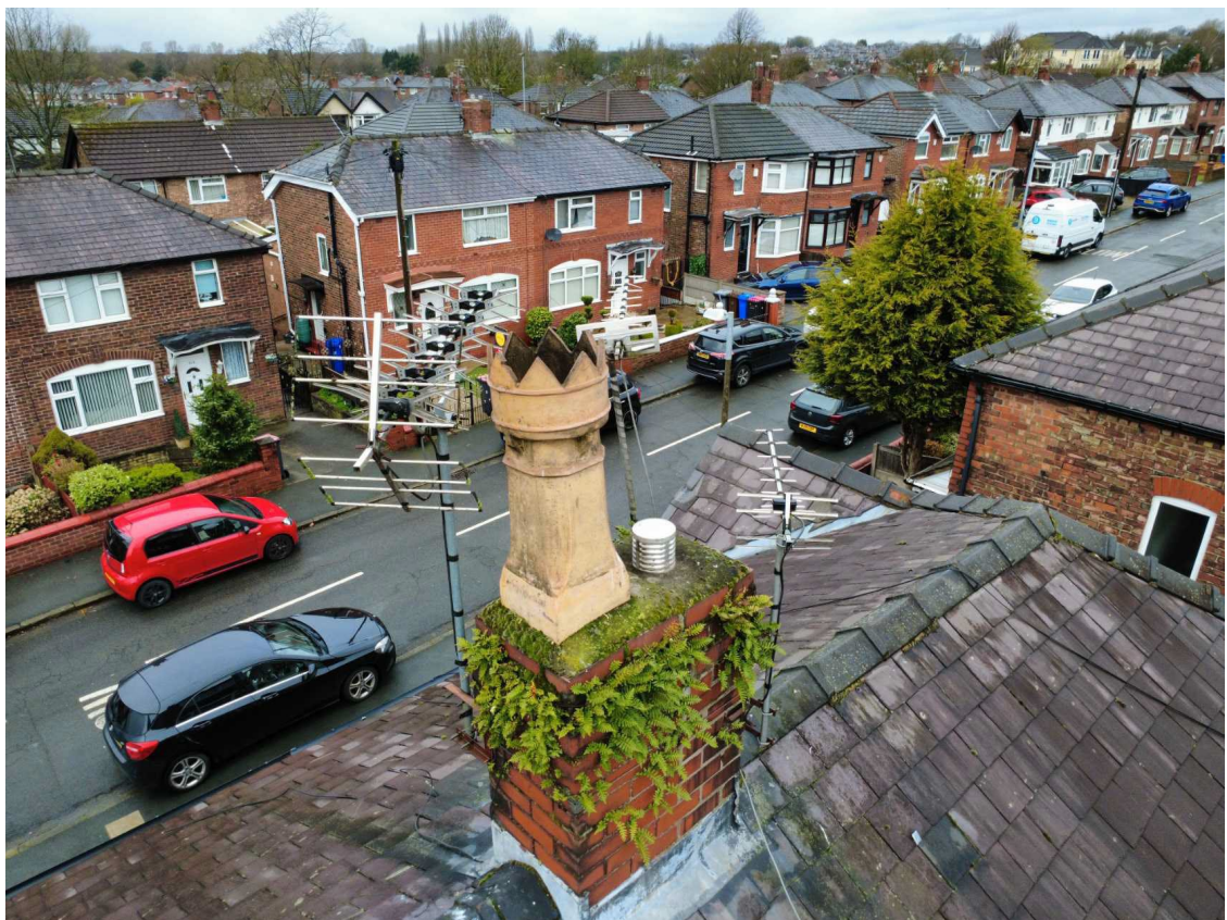
View to chimney flue
