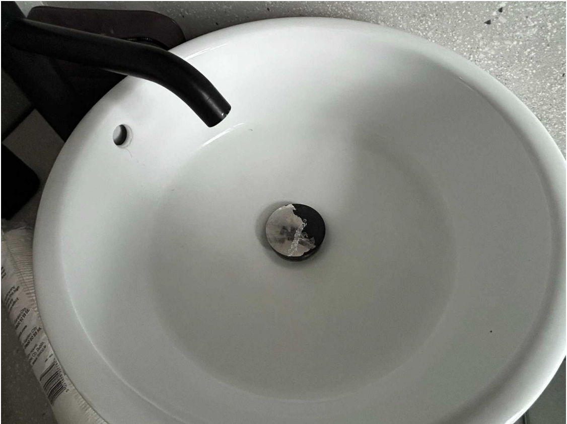
View to the hand basin worn chrome stopper
