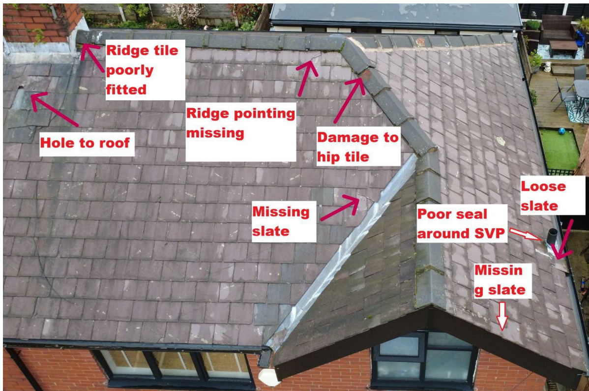
View to main roof from front
