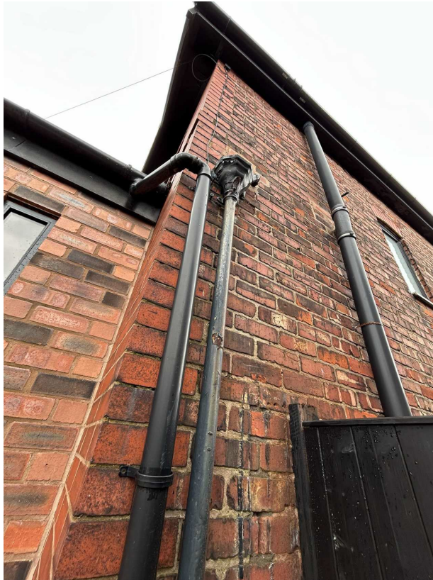
RWP to porch roof
