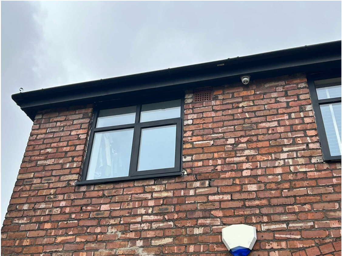
View to rear elevation
