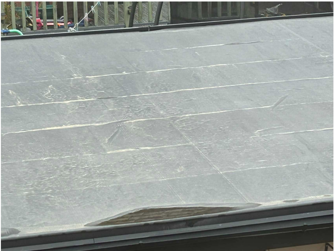
View to flat roof to out building
