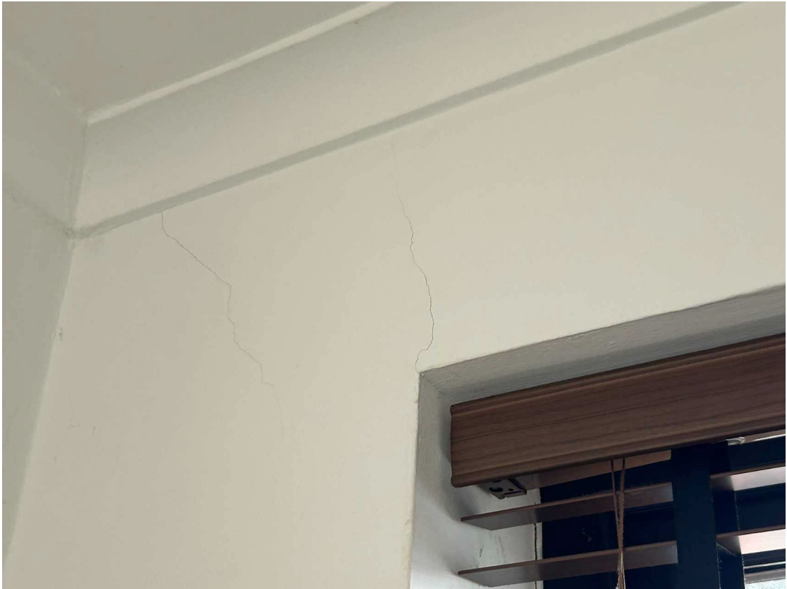
Minor cracking
