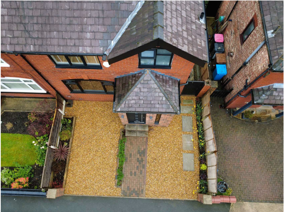
View showing the porch roof to the front
