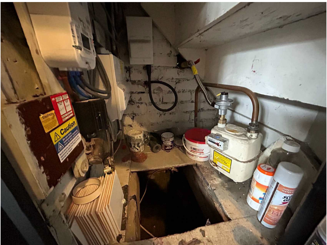
View to access to floor void under the stairs
