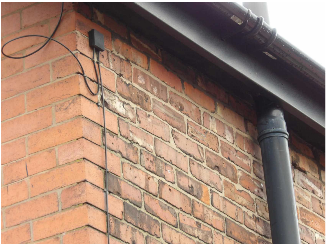
Close-up view of the right hand elevation eaves
