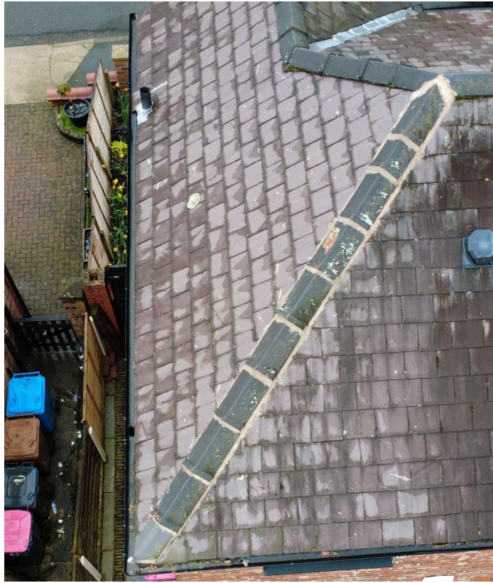
View to gable roof slope
