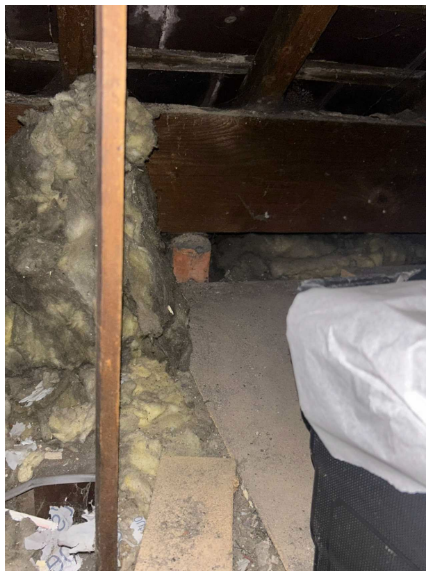
View to front purlin supported of cross wall
